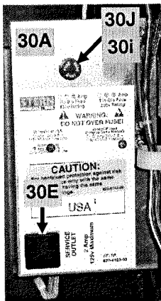
Enlarged Inside Cabinet View of Items 30, Power Box (30A), Service Outlet (30E), Fuse (30i) and Fuse Holder (30J).
